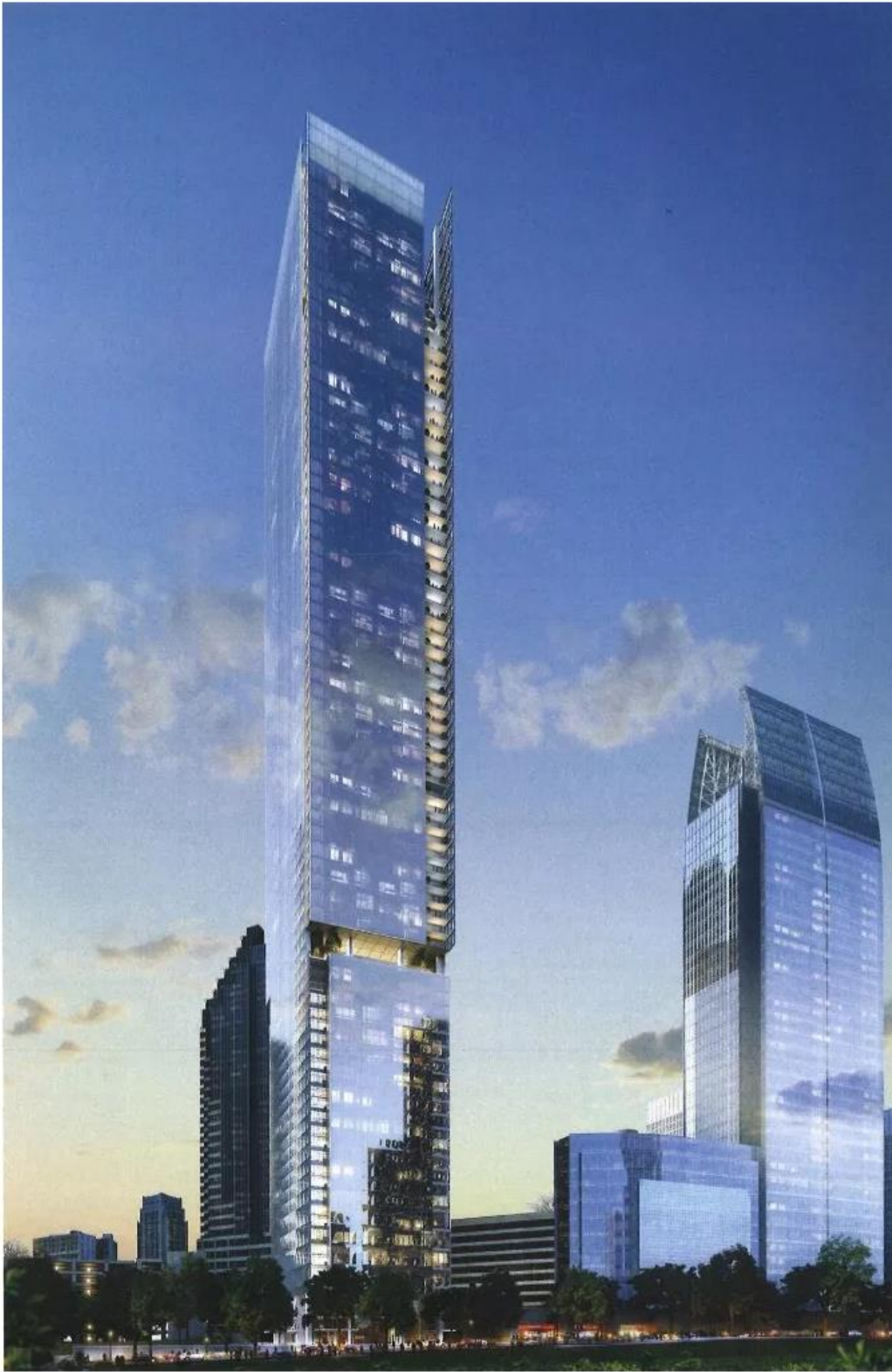
A view of No2 Opus. | Perkins + Will
