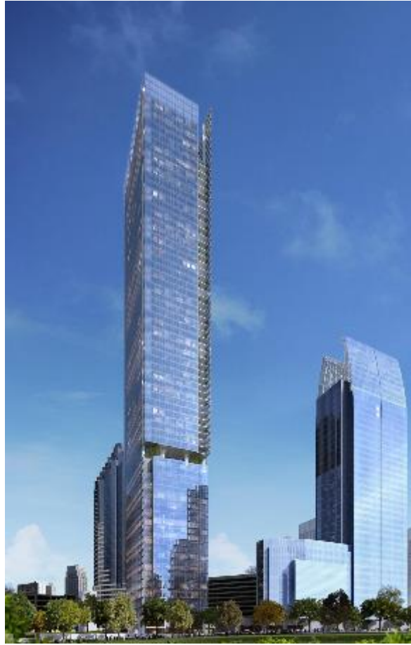
Another view of the new tower proposed by Olympia Heights Management.
